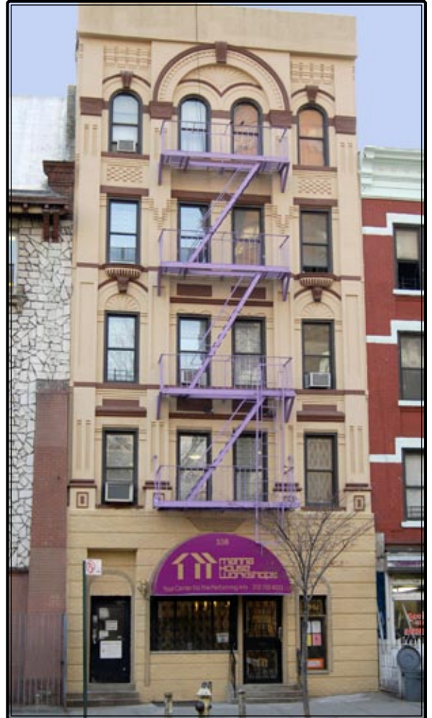
Our newly restored façade
